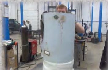
Installing Stainless Steel Housing
