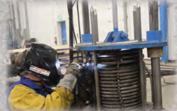
Compressing & Welding Pancake Bracing
