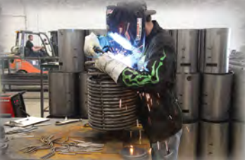
Welding Additional Bracing
